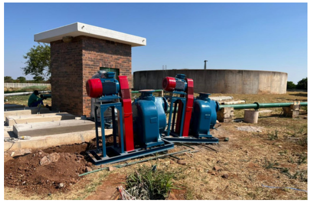
Waste Water Treatment Plant Pump Installation
