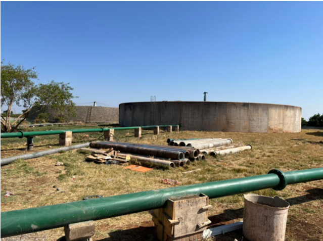
Replacement of Asbestos Pipes
