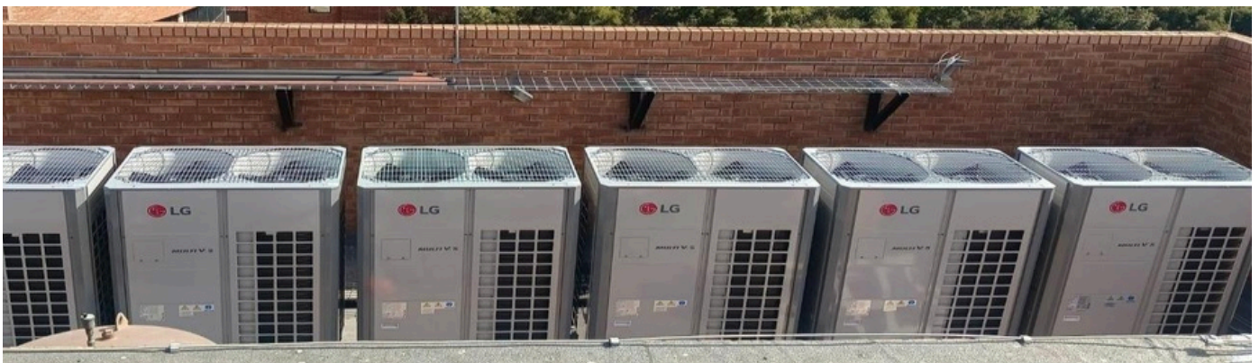
Condenser Installation for HVAC
